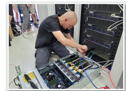
installation of 3rd GPU [19-23/08]
