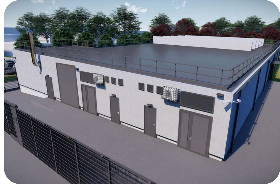
The new RUB data center
